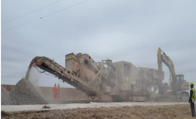
Figure 2: Site review of crushing plant
