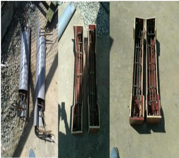
Figure 5: Formworks for various columns
