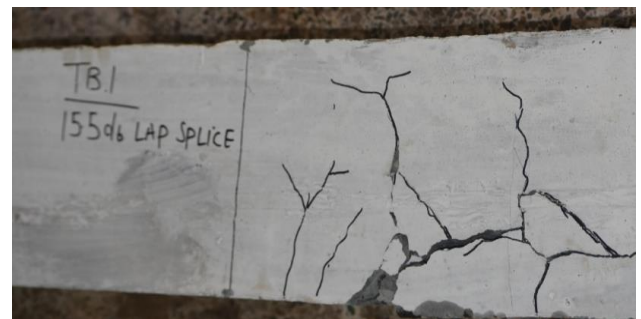
Figure.4: The TB1 crack patterns
