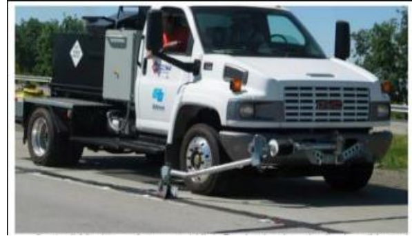
Figure 1: crack sealing
