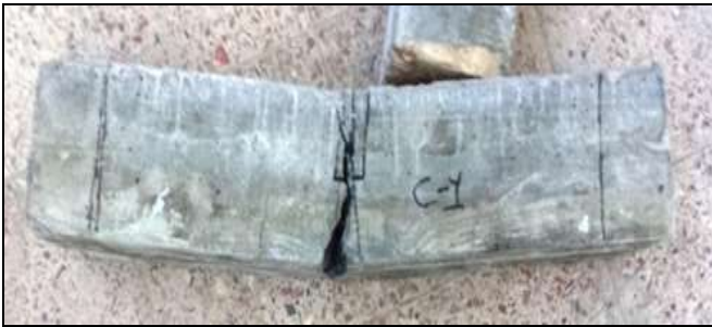
Figure 9: Failure Photo of Beam C-1
