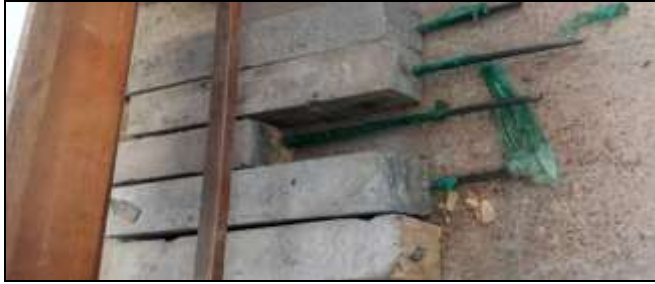
Figure 4: pipes casted in the bottom surface of the beam
