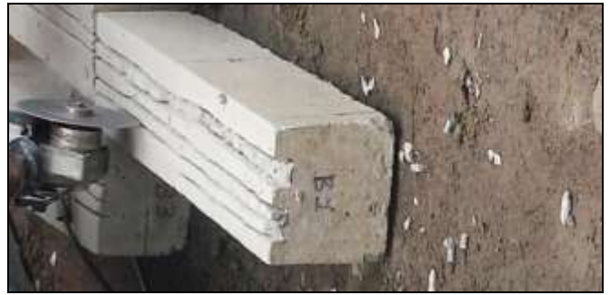
Figure 2: Groove preparation saw cut and chiseled
