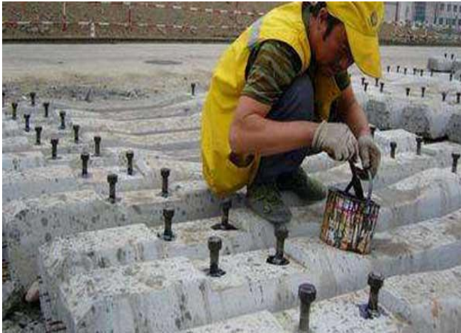
Figure 7: The Procedure for Securing a Railroad Spike to a Railway Sleepers.
