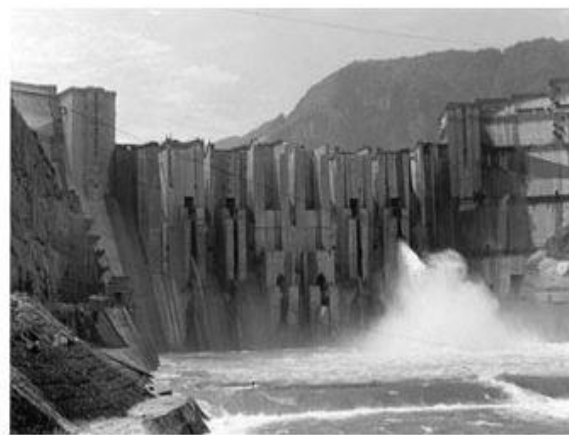
Figure 1: The above figure shows the Slit Bucket at Geheyan Dam in China
