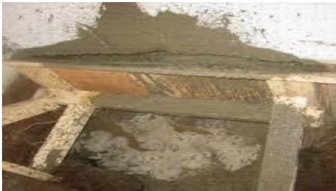
Figure 7: Dry packing of concrete
