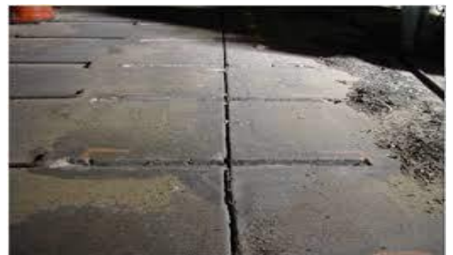
Figure 6: Stitching of Pavement
