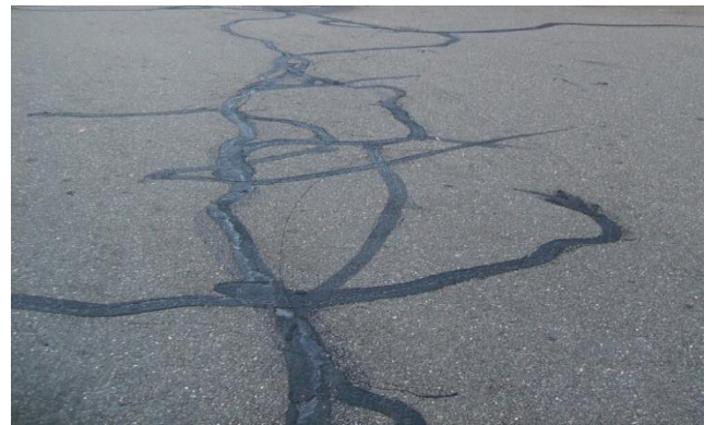
Figure 5: Routing and sealing
