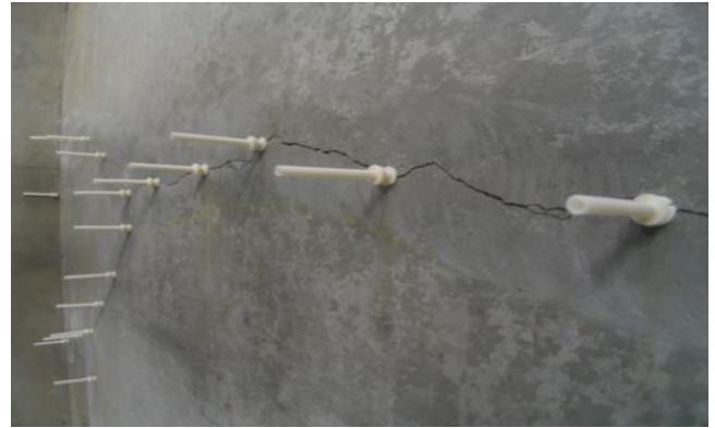
Figure 4: Epoxy injection in cracked wall
