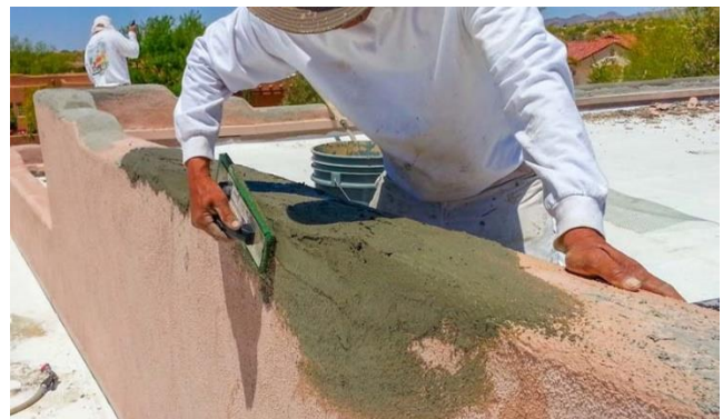
Figure 2: Repair of Parapet wall
