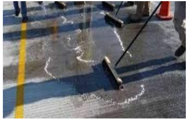
Figure 8: Polymer impregnation of a road
