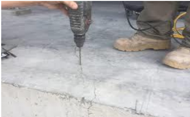
Figure 6: Drilling & plugging in cracks
