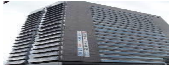
Figure 9: Kyocera Headquarters in Tokyo Japan with BIPV
