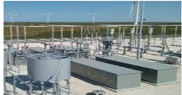
Figure 5: Capacitor banks for a wind farm
