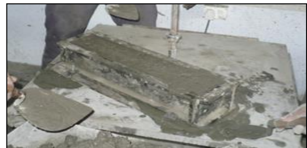
Figure 3: casting of beams
